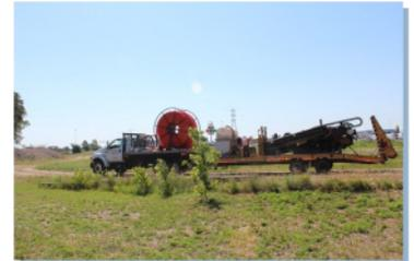
where the running line of the fiber path is obstructed. Examples of obstructions in the running line include trees, rivers, streams, roads and railroads. Once the bore is completed by drilling a hole with metal pipes and a drill head, the conduit is then pulled back and “placed” through the hole.
