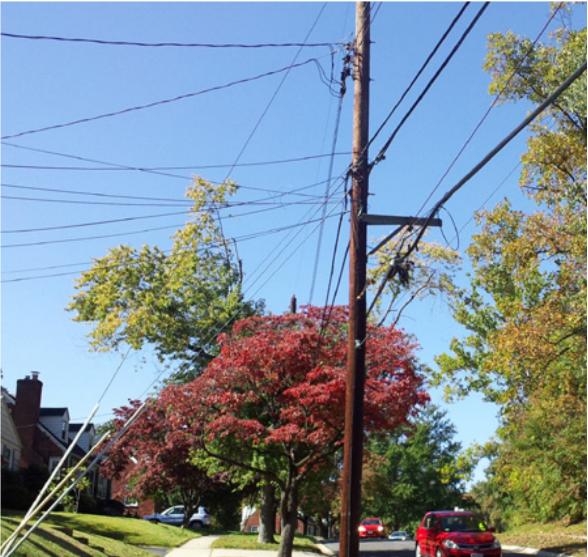
FIGURE 20: EXAMPLE OF EXTENSION ARM ON POLE, ENABLING HORIZONTAL EXPANSION OF CAPACITY
